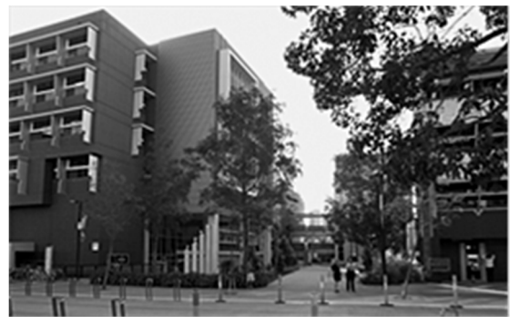
TAFE Queensland South Bank Campus
